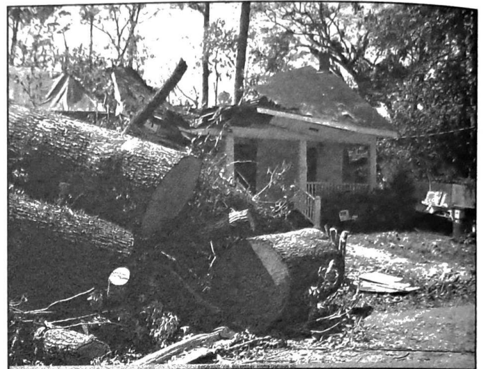
Damage from Katrina
